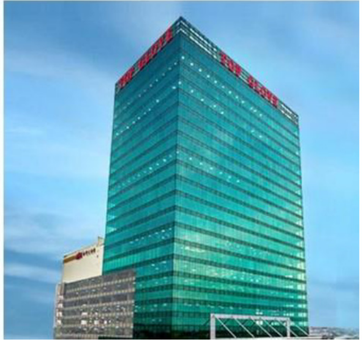
Top Glove Tower Project
